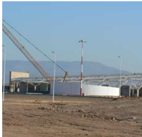
Work on Oujda Airport's second terminal (35 minutes drive from Saïdia)
