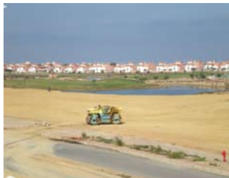
Ground works complete on VVT-4
