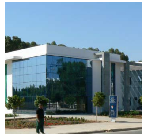
New office buildings being developed in Saïdia
