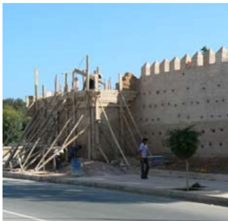
Restoration of the 16th Century Kasbah in Saïdia
