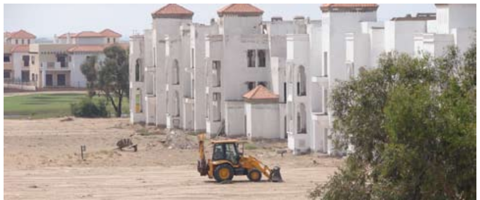
Landscaping preparation on RT-2
