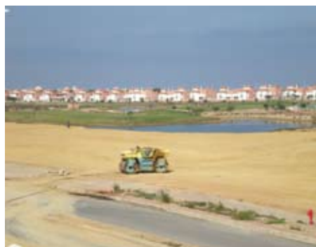
Ground works complete on VVT-4
